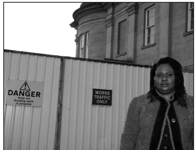
Councillor Sharon Hamilton standing by the protective barriers still surrounding the Mansion after more than four years. In spite of some work having been completed, there's still no sign that it will be re-opened soon.
